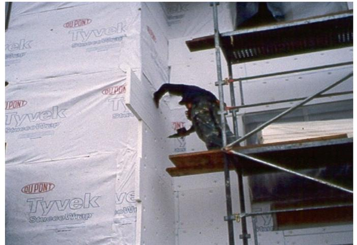
**Figure 3. DuPont™ Tyvek® StuccoWrap® air and water barrier behind exterior polystyrene rigid insulation**
