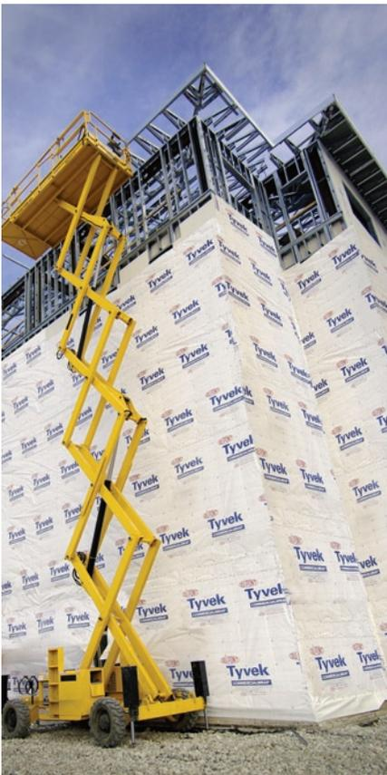
Vapor permeable membranes like DuPont™ Tyvek® CommercialWrap® and DuPont™ Tyvek® StuccoWrap® will perform the air and water barrier functions in exterior insulation wall design.
