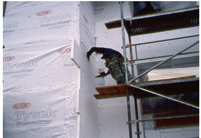
Figure 3. DuPont™ Tyvek® StuccoWrap® air and water barrier behind exterior polystyrene rigid insulation
