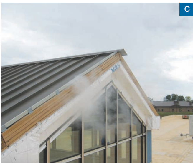
Non-continuous air barrier at roof-to-rake-wall interface. (A) Digital picture; (B) IRT scanning performed under building pressurization; (C) Large-scale smoke tracer generation test performed under building pressurization.
