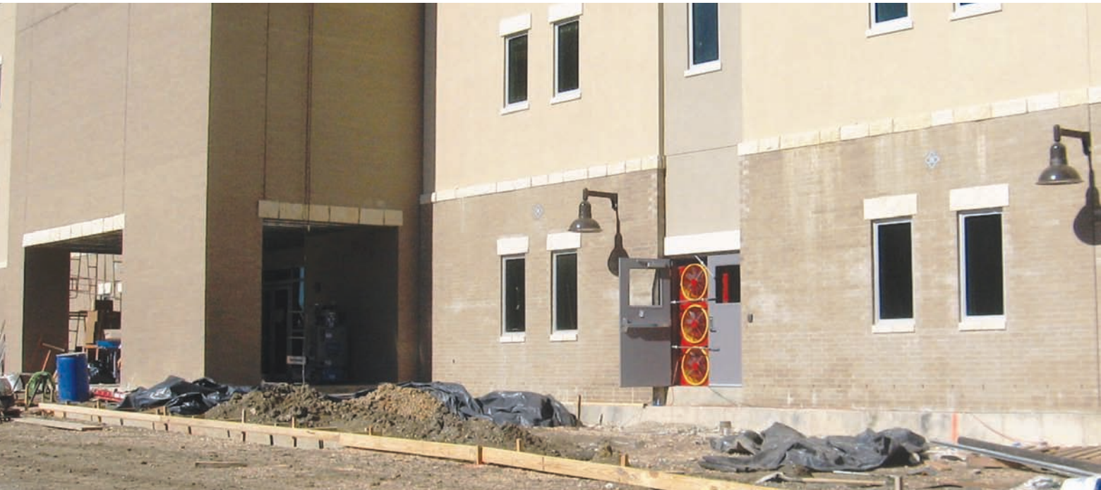
Airtightness testing for a larger building. Multiple three-fan setups are typical for such sizable structures.
