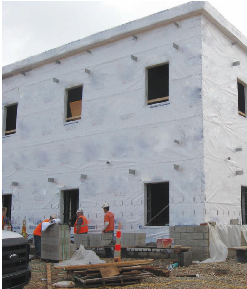
Overview of mechanically fastened sheet air barrier system installation.
