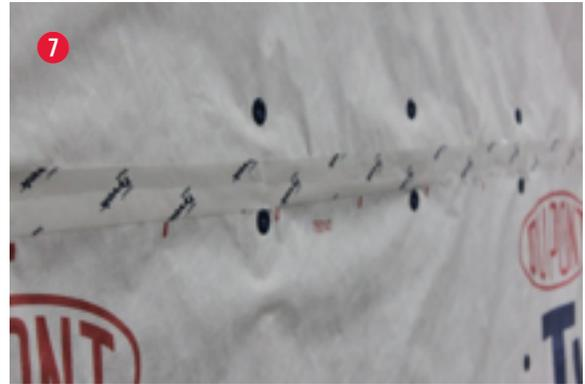
5. Install the second layer of **DuPont™ Tyvek® WRB** maintaining a 6" minimum overlap with first layer. Tuck edges tightly into sealant and corners of framing as shown above. Use firm hand pressure or j-roller to ensure a positive bond to sealant. Cut excess **Tyvek® WRB**.
