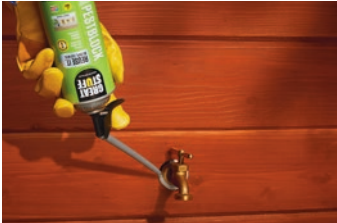
Water Faucet Penetration
