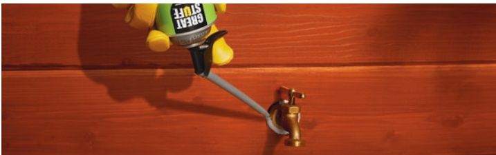
Water Faucet Penetration
