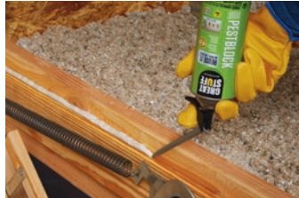
Attic Hatch Frame
