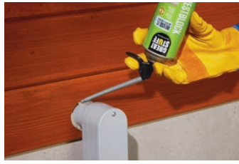
Electrical Cable Lines
