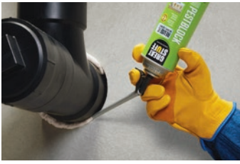
PVC Pipe Penetration
